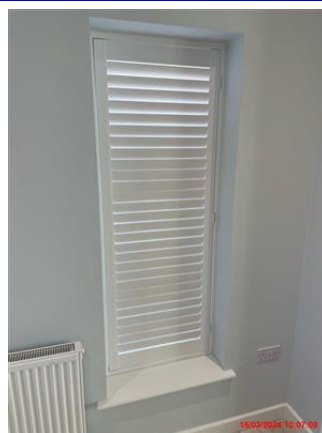
White wooden double fold plantation shutters. Well fitted. Slightly dusty but in good condition.
