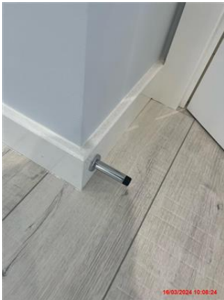
White painted skirting boards. Woodwork and paintwork in good condition. Chrome doorstop with black tip - intact.
