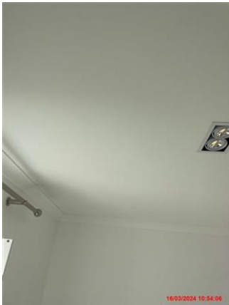
White painted ceiling. Ceiling and paintwork in good condition.
