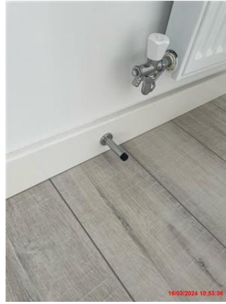
White painted skirting boards. Woodwork and paintwork in good condition.
