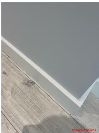
White painted skirting boards. Woodwork in good condition. Slightly dusty at the tops.
