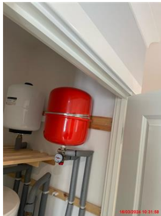
White painted door frames. In good condition.
