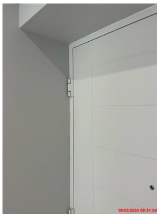
White painted door frames. In good and clean condition.
