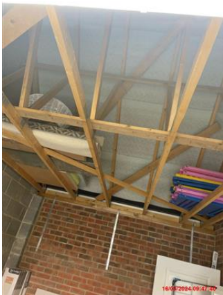
Wooden beam construct. Beams intact and well fitted.
