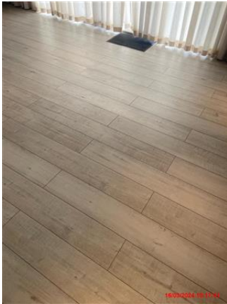
Grey laminate flooring. Floorboards intact. In good and clean condition.
