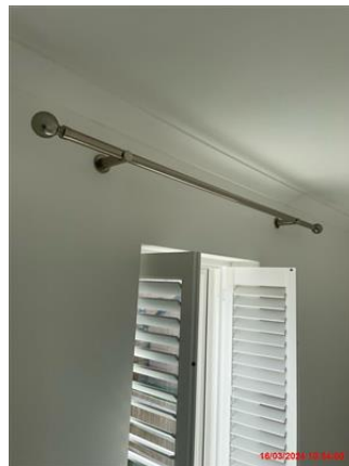
Chrome curtain rail fitted to wall above window. In good condition.
