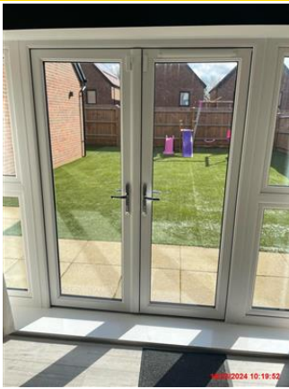
White UPVC doors. Chrome handle - intact. Double glazed. Doors sturdy. Secure. In good and clean condition.
